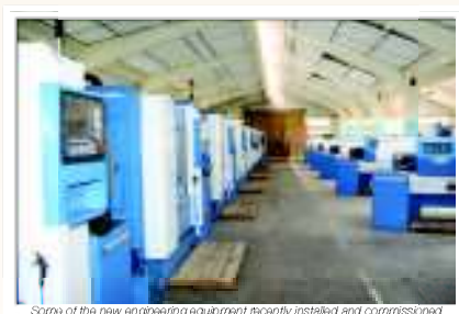
Some of the new engineering equipment recently installed and commissioned
